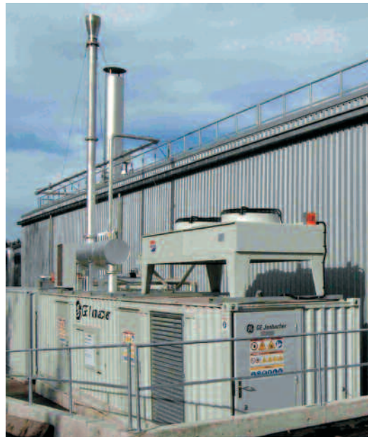
Fig 3 Typical containerised CHP unit for biogas
