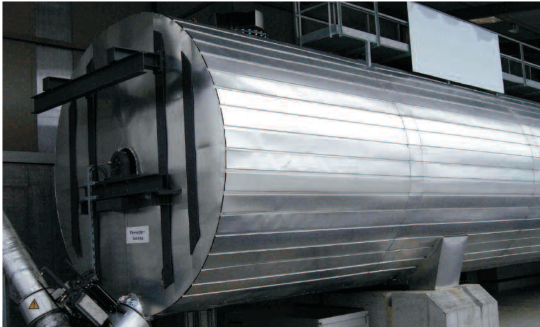
Fig 4 Anaerobic digester suitable for treating 5,000 tonnes/year of biowaste (including food)
