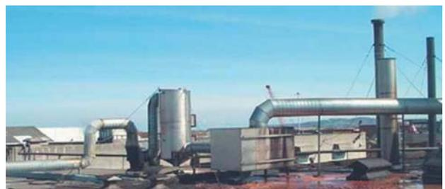
Figure 2: Air scrubber and cooker exhaust stacks
