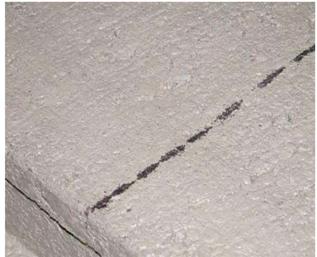
Fig 4. Slabs marked for cut out.
